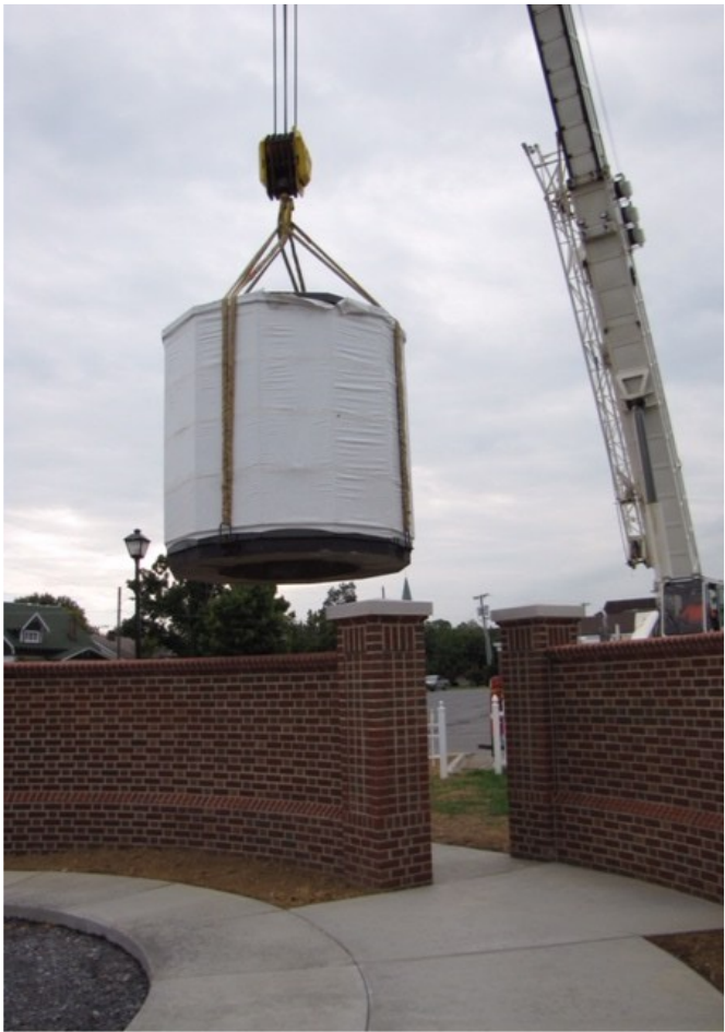
The vault of the columbarium which contains the individual niches is lowered into place
