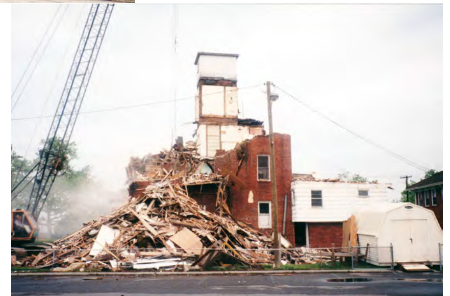
Right: McNeer Building Demolished in 1996
